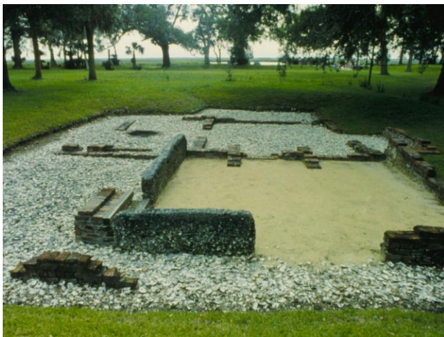
Figure 2. Foundations to the Hawkins-Davison Duplex. The Davison structure is in the foreground.
