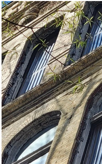
Figure 15. Arched Lintel with Key Stone
