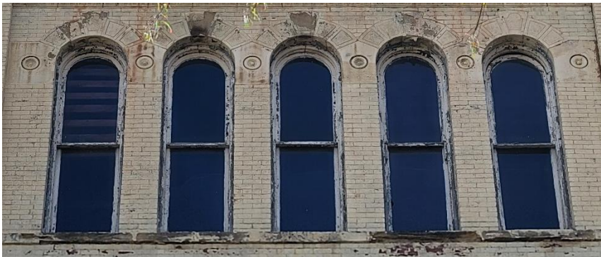
Figure 21. Arched Lintel with Keystone
