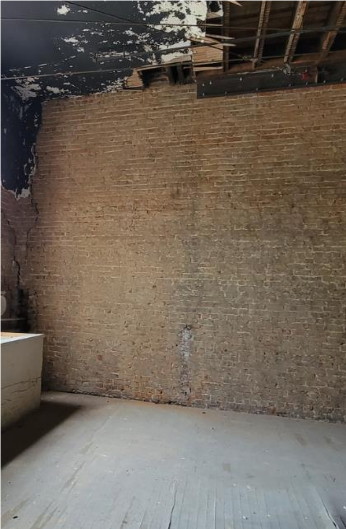
Figure 28. The Current State of the Structural Brick Wall
