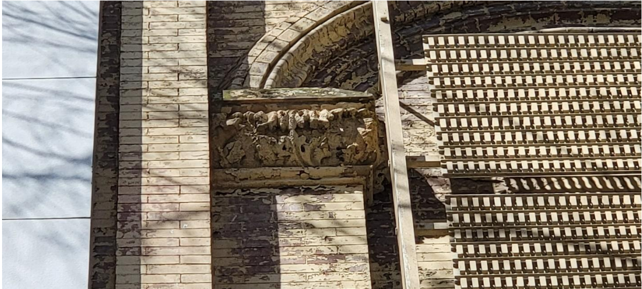
Figure 13. Pilasters Topped with Romanesque Capitals
