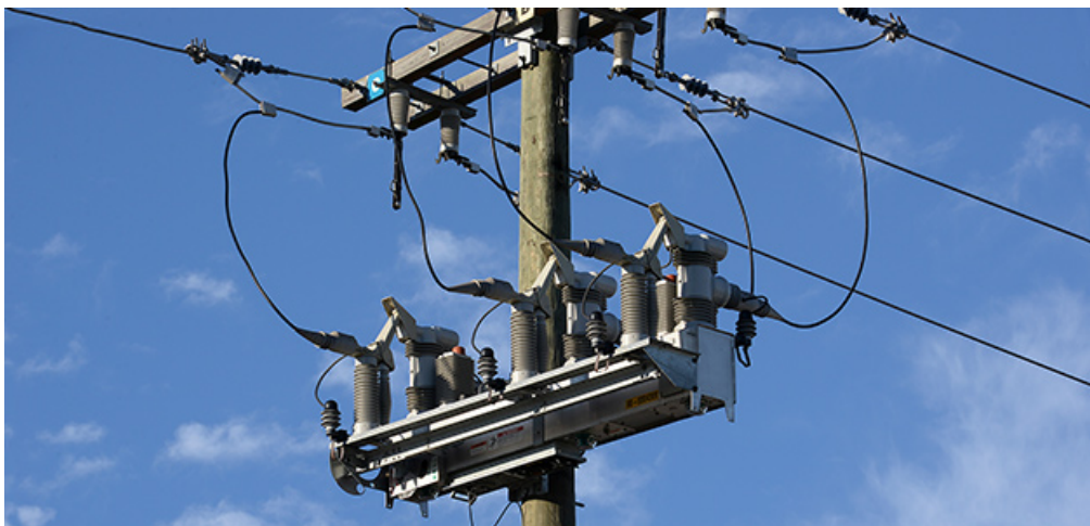
Figure 1 S&C IntelliRupter ® PulseCloser ® Fault Interrupter [1]
